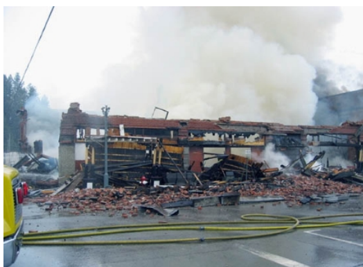
Figure 1.3: A hotel building damaged by fire
